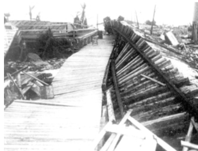
Destruction of the Florida East Coast Railway in the aftermath of the storm
