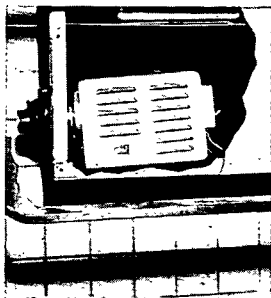
Four Dage Closed-Circuit TV Cameras like this one are mounted at spaced intervals on the ceiling of the Turnpike tunnel. Each feeds signals to its own Dage receiving set in the control room at one end of the tunnel.
