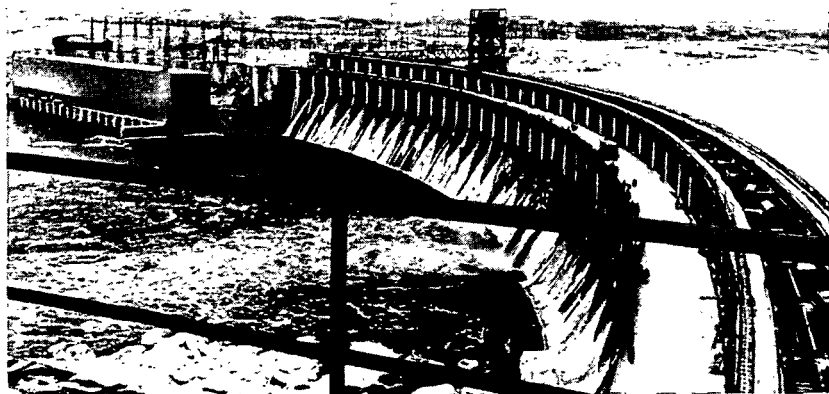
A government project that literally blew up—the Dneprogez dam.
